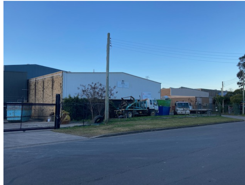
PHOTO 2: Looking north from street to 29 Plasser Crescent
